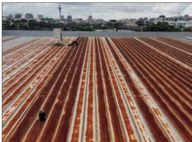
Roof refurbishment in Auckland (Jotamastic).
