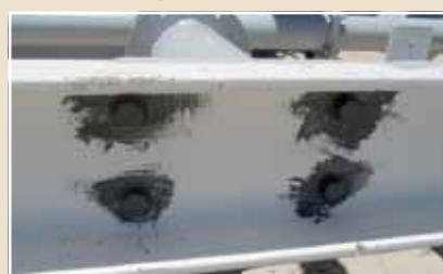
Zinc electroplating coating thickness 26µm.
