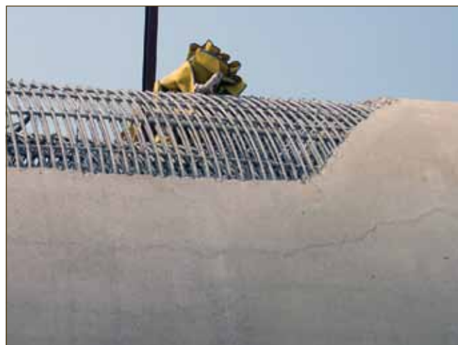
Changi outfall pipes, Singapore.
