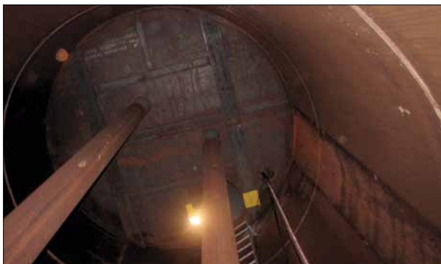
The sealed portion of the monopile below the lower platform.
