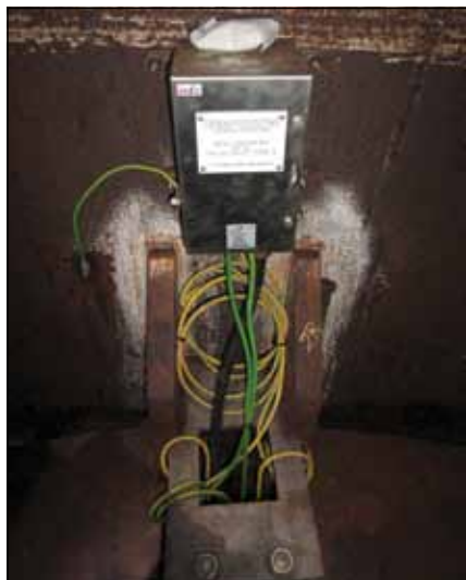
The junction box, installed above the lower platform, connects the anodes to the structure.
