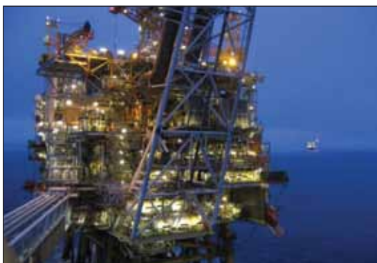
Figure 24: More than 8 000 flanges coated.
