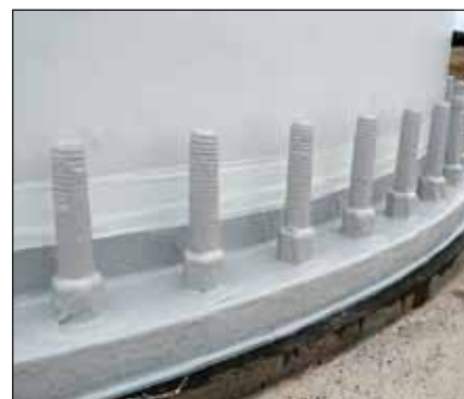
Figure 30: CIST coated bolts on a wind turbine tower.
