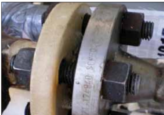
Figure 23: Mixed carbon and stainless substrate after 7 years.
