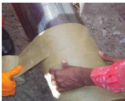
A 55% overlap is ensured during wrapping of DENSO Petrolatum inner tape. This application will ensure long term corrosion prevention.
