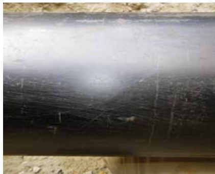
Pipe in an immaculate condition.
