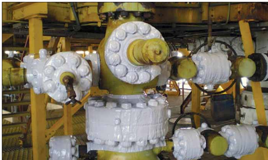
Figure 4: Remedial application to North Sea Wellhead.
