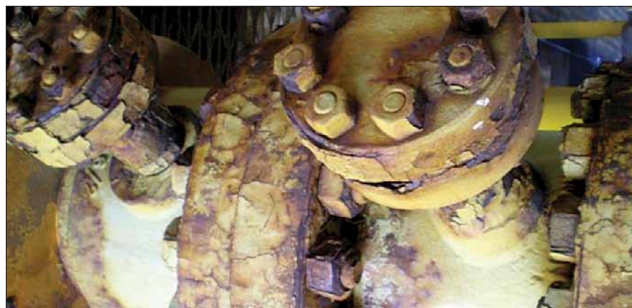
Figure 3: Ageing infrastructure in the North Sea.
