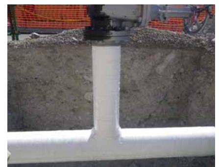
Here we see tie in wrapped with DENSO primer, DENSO petrolatum tape and DENSO outer wrap.
