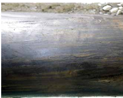
The petrolatum compound has formed a protective layer even after the removal of the DENSO petrolatum inner wrap.
