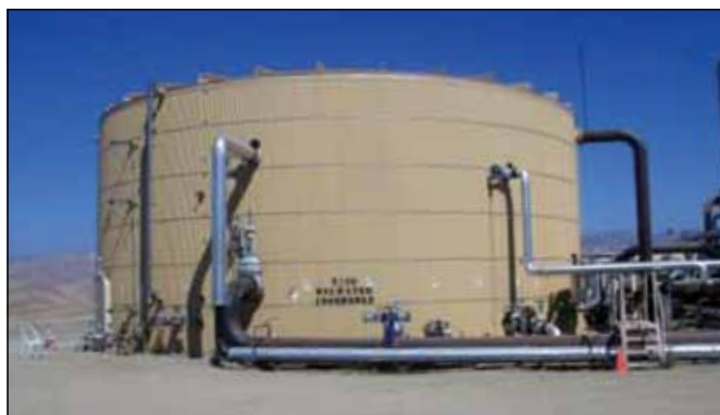
Water is typically accumulated in 5 000- to 10 000-bbl (795 000 - to 1.59 million-L) produced water tanks.
