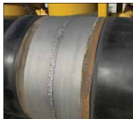
A close up of a welded and repaired field joint.
