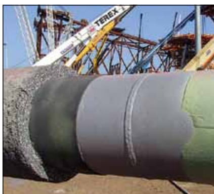
Field joint on riser.
